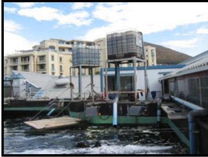
Figure 3: Flushing devices and water movement systems at the Cape Town Aquarium
